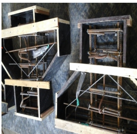
Plate 1: steel reinforcement of corbel
