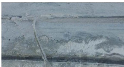
Plate 3: Putting CFRP inside groove with epoxy paste adhesive
